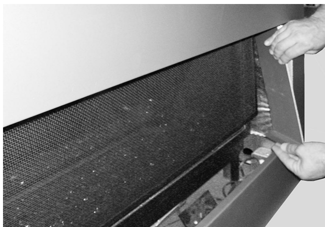
STEP 5: Insert the right side panel into the opening angling in at the top.
