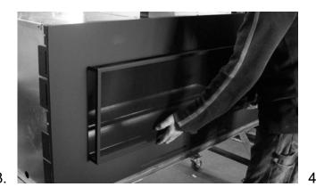
Rotate the bottom of the screen inward and position the center tab into the notch on the fireplace tray. Bottom side tabs should rest inside the firebox opening.
