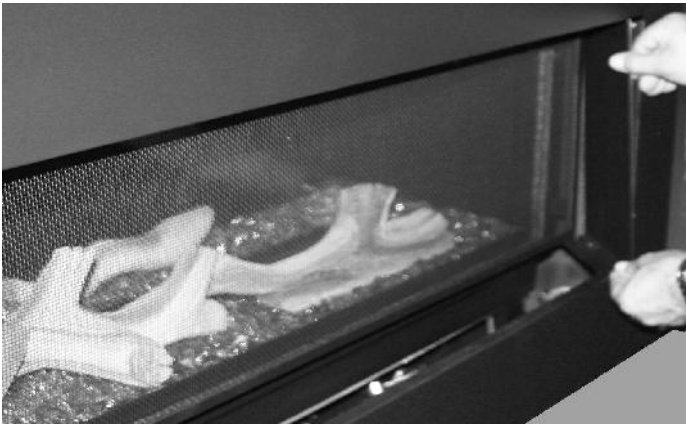
STEP 5: Insert the right side panel into the opening angling in at the top.
